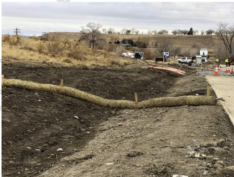
Fig. 13 Photograph of straw wattle used to control soil erosion during construction.
