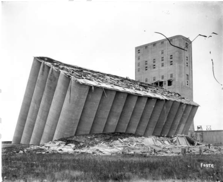
Fig. 5 Transcona silo bearing capacity failure (Manitoba Historical Society, 2018).
